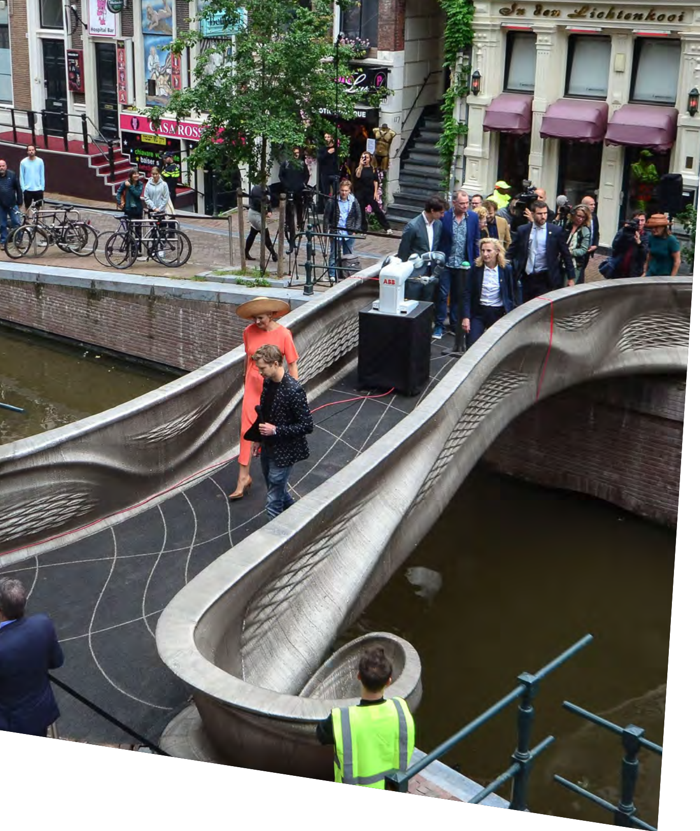
The world's first 3D printed steel bridge was opened by Queen Máxima of the Netherlands in Amsterdam in July 2021
